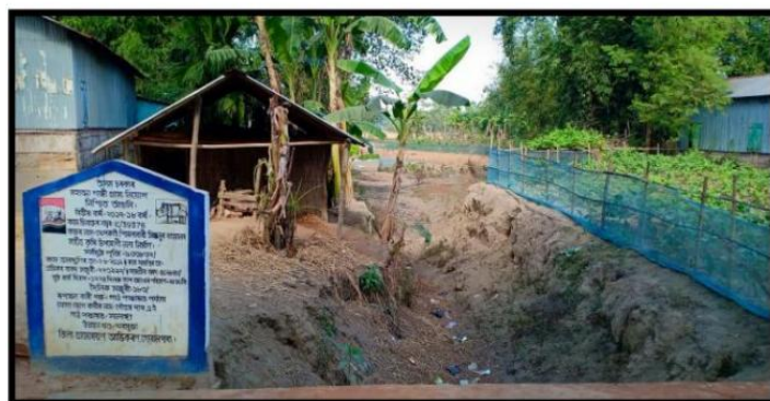
BEFORE COMMENCEMENT OF WORK
